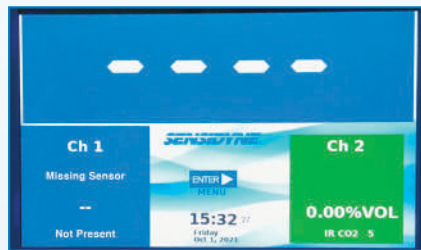
CH-1 Fault CH-2 All Safe
